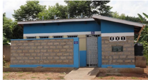
5 stance VIP latrine with a urinal for boys and bathroom, incinerator for girls, constructed at Ikumbya Catholic Primary School in Luuka District
